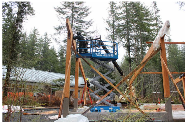
Construction crews are making good progress on the education pavilion.
